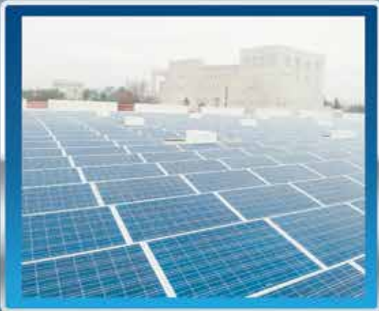
On Grid , Off Grid
